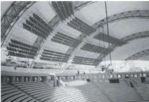
Figure 9 – Interior view showing the sound absorptive panels at the rear zone of the amphitheatre
